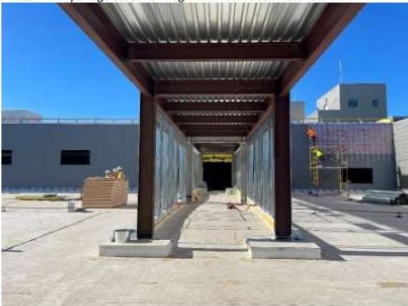
Photo 7 – Skybridge steel framing with metal deck installed.
