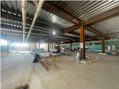
Photo 7 – Skybridge steel framing with metal deck installed.
